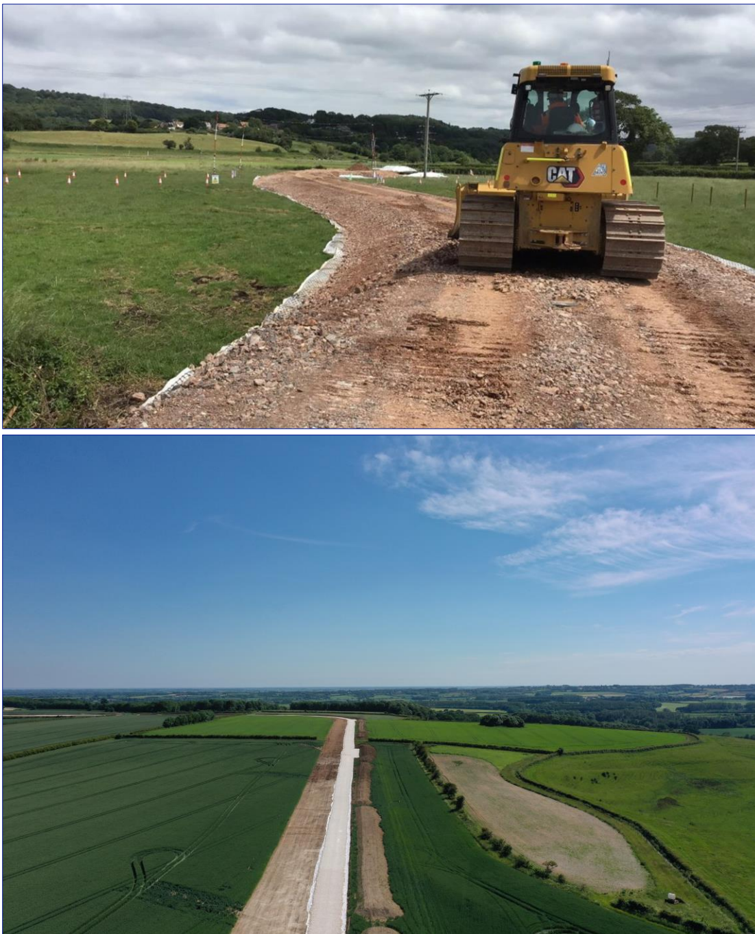
Figure 6.1: Typical temporary access roads constructed with stone
