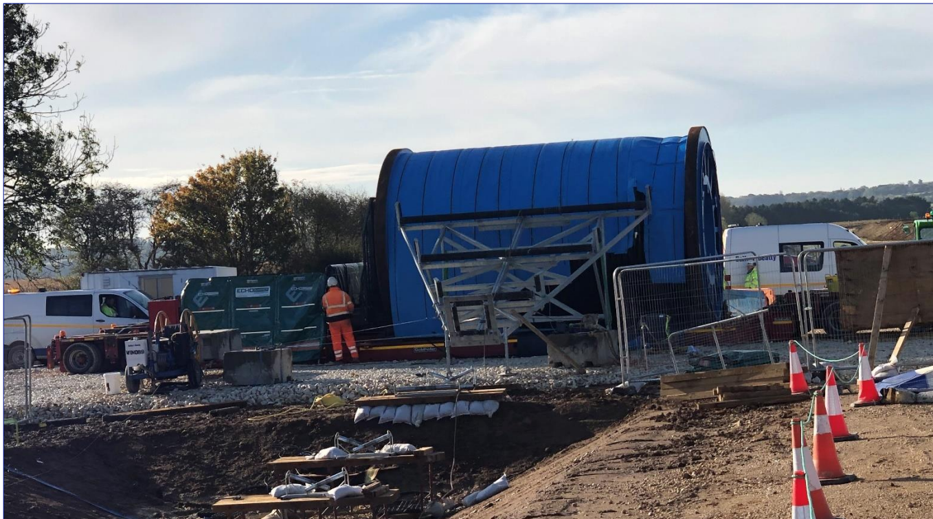
Figure 4.5: Cable Drum Delivered to Site
